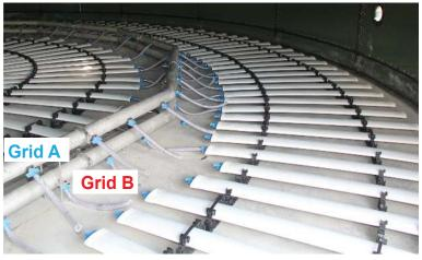
One set of Dual-Air-Control – OxyStrip diffusers equals eighteen 9" disc diffusers
