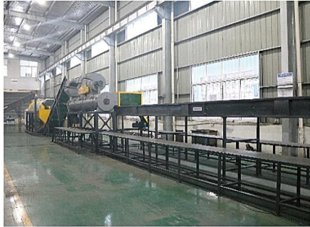
MT-500 PET Washing Line in Poland
