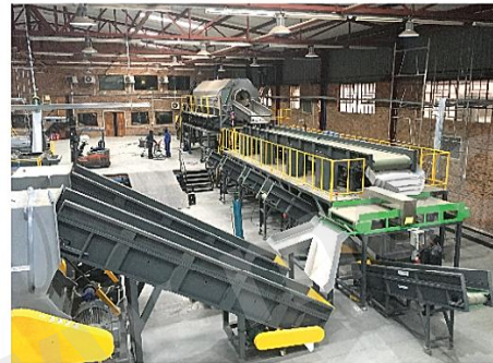
MT-2000 PET Washing Line in Algeria
