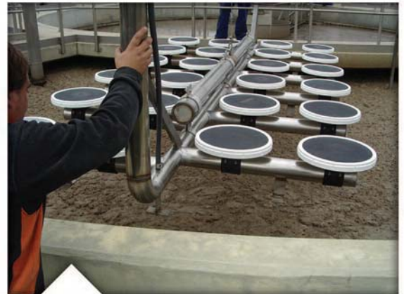
Disc diffusers provide exceptionally high oxygen transfer efficiency in this aeration tank in Spain.
